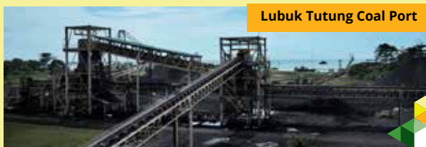
Lubuk Tutung Coal Port Lokasi : Lubuk Tutung, Kalimantan Timur Location : Lubuk Tutung, East Kalimantan Timur Fasilitas : Coal crushing facility, Stockpiling facility & Coal loading port Facility : Coal crushing facility, Stockpiling facility & Coal loading port
