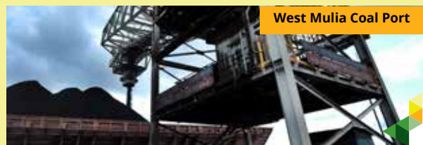
West Mulia Coal Port Lokasi : Desa Mekar Sari, Kintap, Tanah Laut, Kalimantan Tengah Location : Desa Mekar Sari, Kintap, Tanah Laut, Central Kalimantan Fasilitas : Stockpiling facility & Coal loading port Facility : Stockpiling facility & Coal loading port
